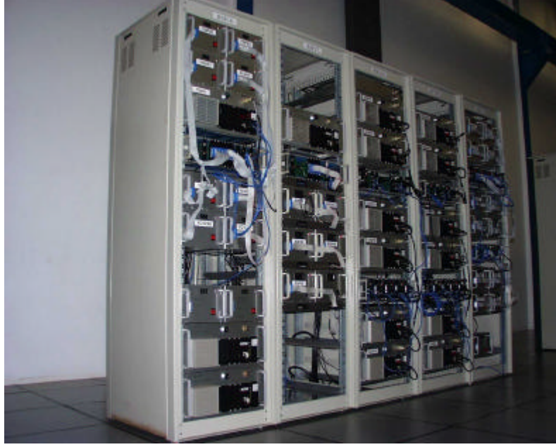
Fig.1 Final installation of the low power current supplies.
