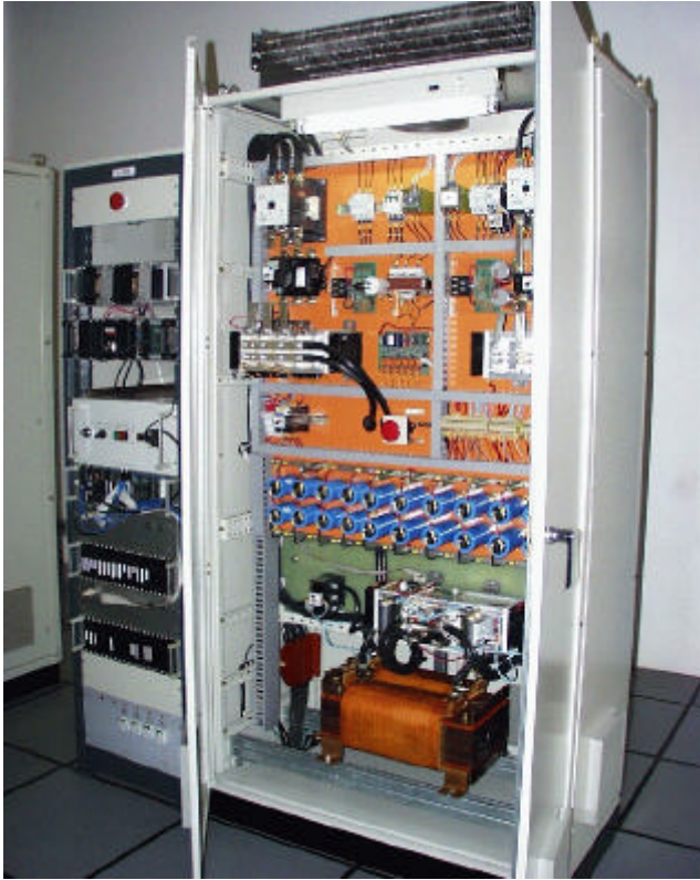
Fig. 10: Front view assembly of the 12-dipole booster power supply, showing the control rack, the thyristor bridge and its LCR filter.
