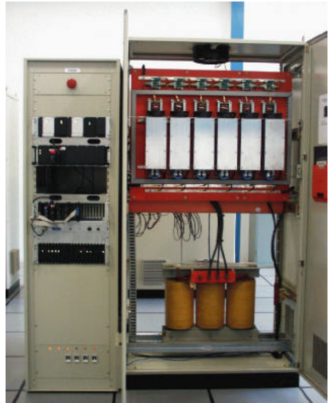
Fig. 13: the 2-dipole current power supply of the extraction transport line.
