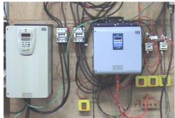
Fig. 11. Variable speed drive with vectorial control and AC-DC converter.
