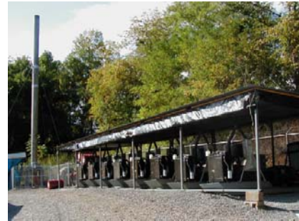
675 kW Synchronous Skid-Mounted Generator sets at Nelm's No. 1 Mine, Ohio (Photo courtesy Northwest Fuel Development, Inc. and U.S. DOE)
