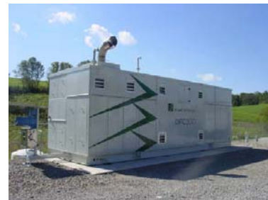
FuelCell Energy DFC Power Plant Installed and Operating Hopedale, Ohio Test Site
